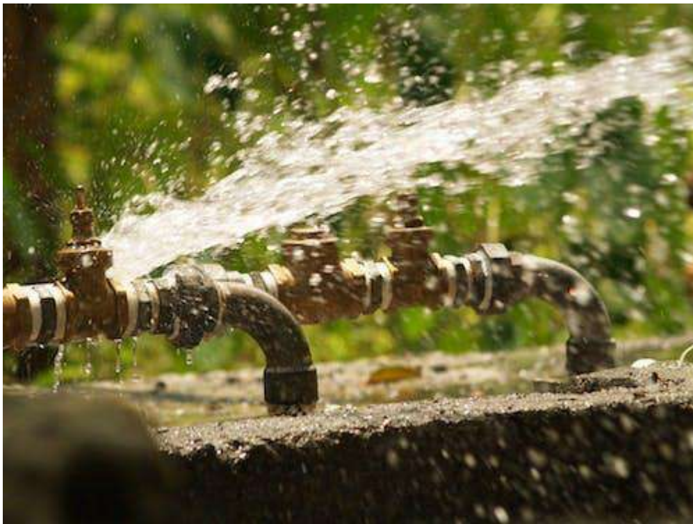
Figure11.2: Typical leaks at a joint
